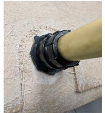
13. Apply provided lubricant **halfway up the tailpiece** and position the bathtub and tailpiece **in line** with the Drop-In Drain.
