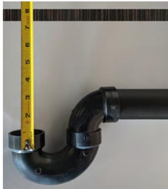
3. Cut the ABS or PVC 1 1/2" pipe 3" shorter than the distance between the floor and the P-trap.
