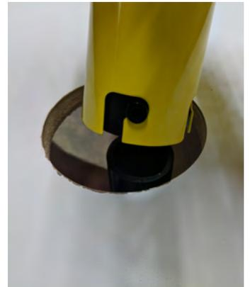
7. Insert the Drop-In Drain cap **firmly** into the Drop-In Drain.
