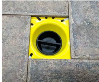
10. Remove the Drop-In Drain cap with a **channel lock plier**.
