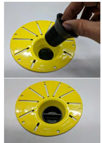
8. Secure the Drop-In Drain to the subfloor with **screws** or **cement**.
