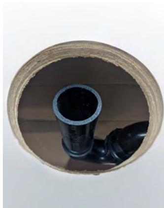
5. Apply glue to the outside of the ABS or PVC 1 1/2" pipe and to the inside of the Drop-In drain insert.
